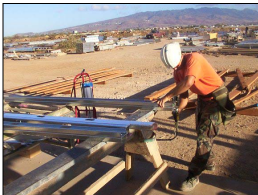
Left: The height of the bench required the user to bend forward and squat downward slightly while trying to position the clinching tool. Right: A framer uses his body weight to apply pressure to a screw gun.
