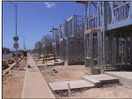
Steel-framed homes under construction at Ocean Pointe.
