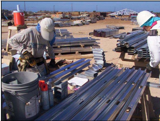
Left: Laborers fabricating panel components off-line. Also, the table height is set for optimum performance with screws. Right: Stud to track assembly under study.
