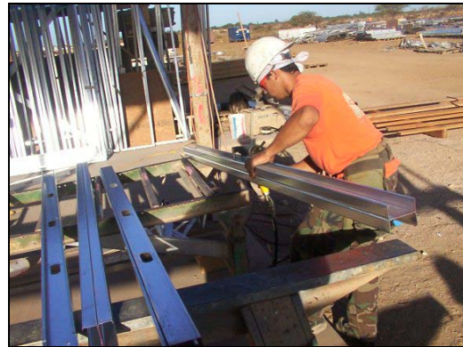
Laborer lifting the studs to slide the clinching tool past table supports. This requires him to hold the clinching tool with one hand and leads to tiring of the arm.
