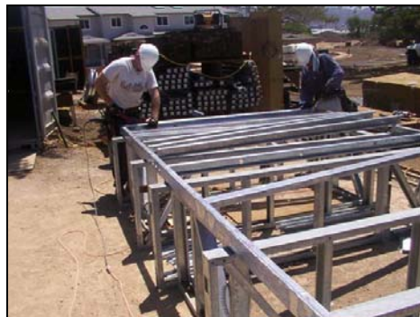
Wall panels under assembly at S&G facility.
