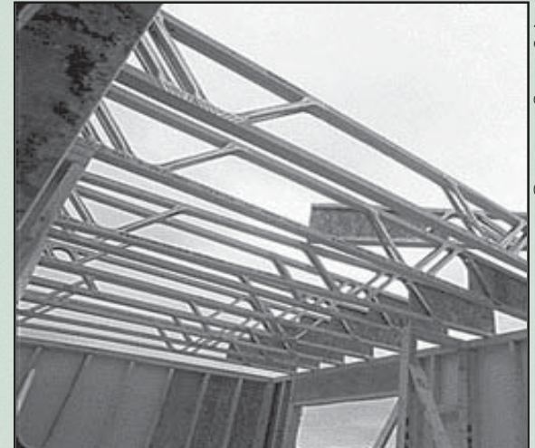
Trim-able Floor Trusses are a hybrid of truss and I-joist technology.
