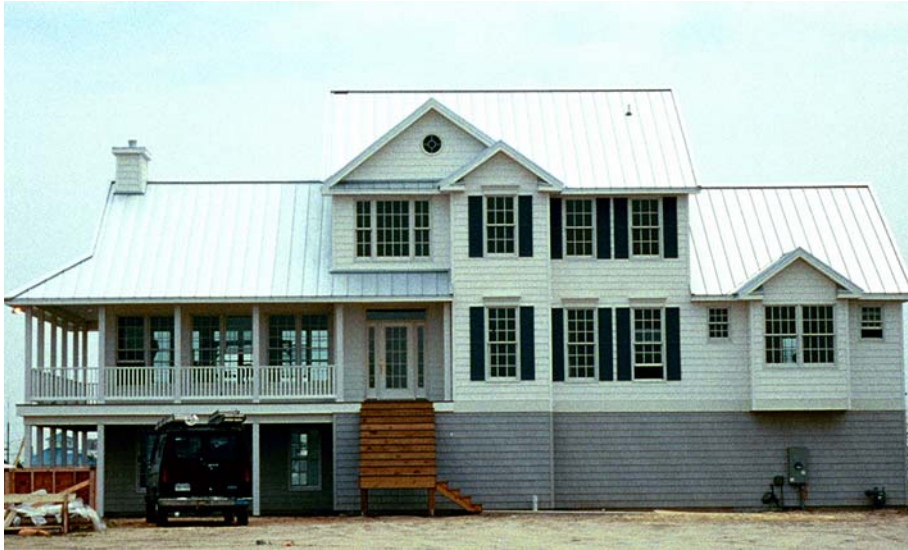
Figure 3 – Cool roof. Photo courtesy of ATAS.
