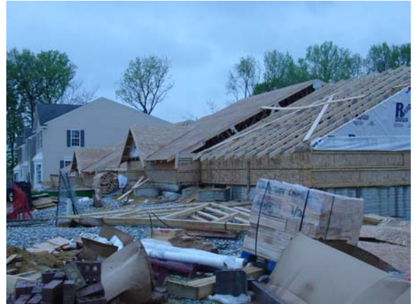
Figure 6 – Ryan Homes Project in Maryland
